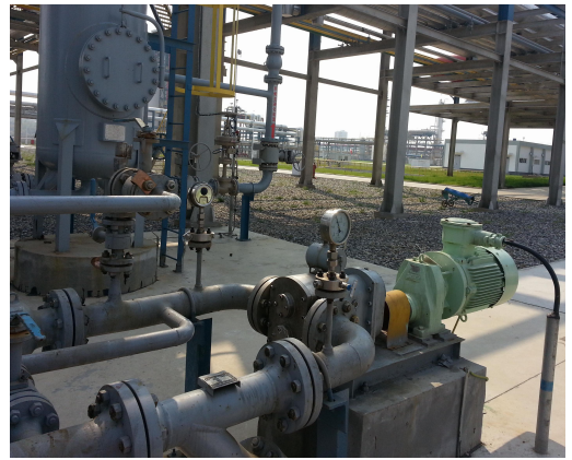
Cam rotor pump for petrochemical plant
